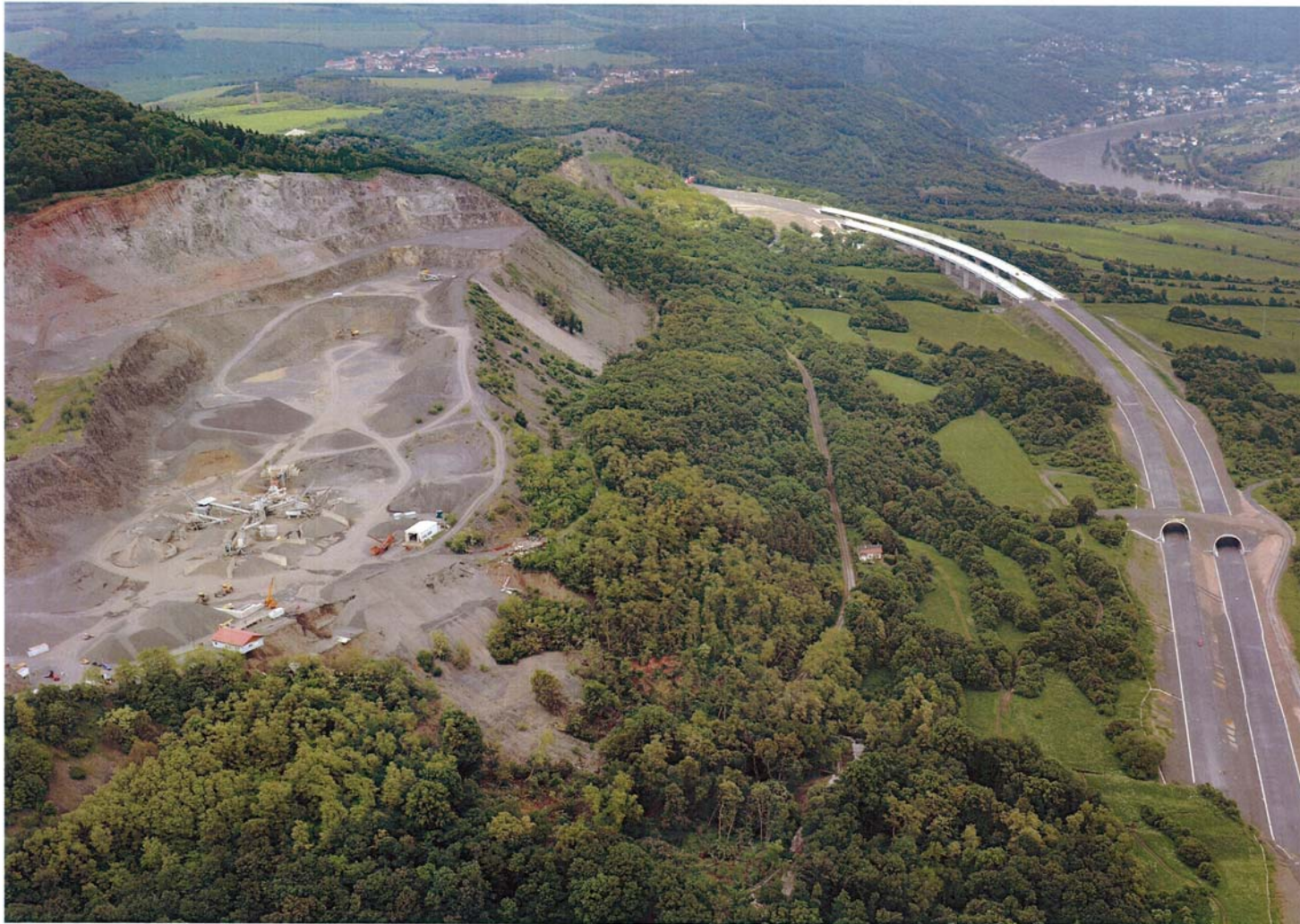
Elbe valley near Prackovice with quarry, railway line and motorway construction site
